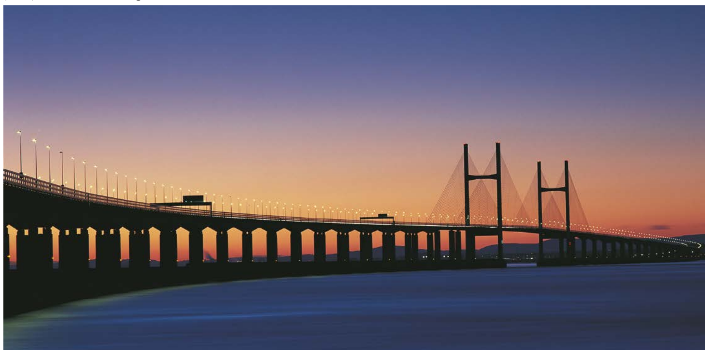
(below) Second Severn Crossing
