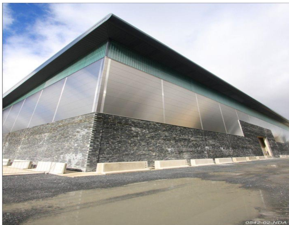
Figure 1: The intermediate level radioactive waste store at Trawsfynydd
